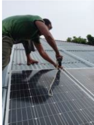
Picture 4. Panel installation on a galvanum frame
